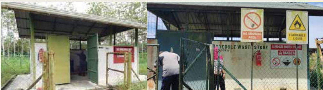
Scheduled Waste Store
