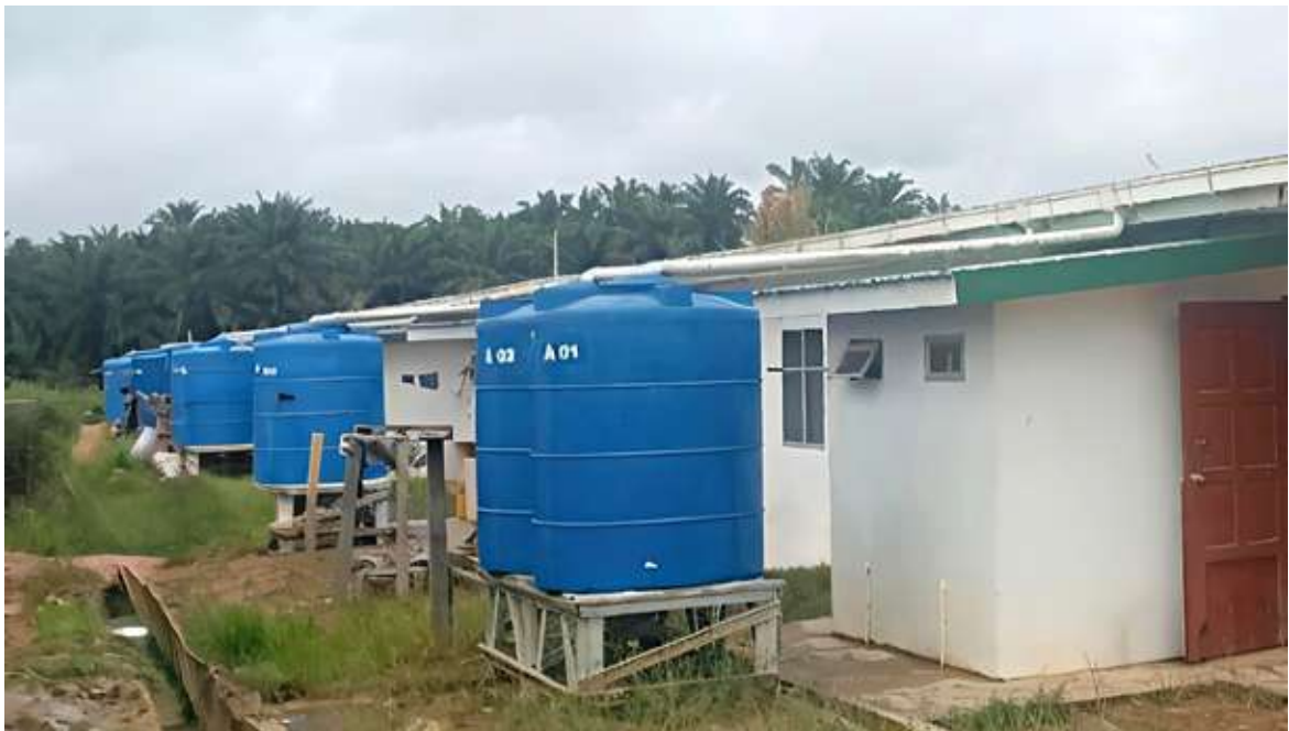
Rain water harvesting tanks
